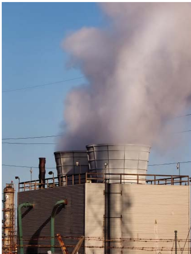
▲ Figure 3. In a counterflow cooling tower, air travels upward through the fill, opposite the downward path of the water.
