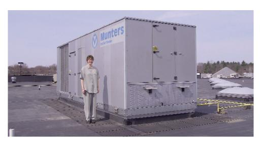
2. Target Air Approach – Some stores have a high concentration of refrigerated cases and benefit from the warm dry air directed in that zone. The majority of the stores ventilation air would be processed through this unit, with multiple rooftop packages serving the general merchandise area.
