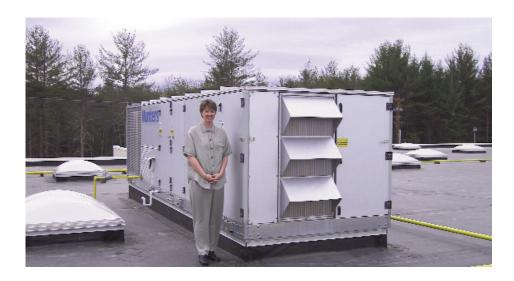
3. Treat Outdoor Air Separately – The third method would be a dedicated outdoor air unit ducted either directly into the space or into a return air duct of either a central system or multiple roof top packages.
