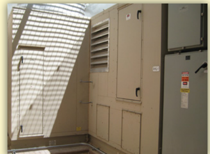
The OASIS systems allow for part (or all) of the cooling requirements of the building to be met without refrigeration.
